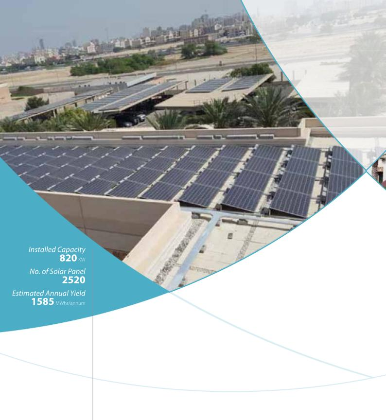
Solar PV panels installed at PIC Head Office Building Roof-top and Car Park Area.
